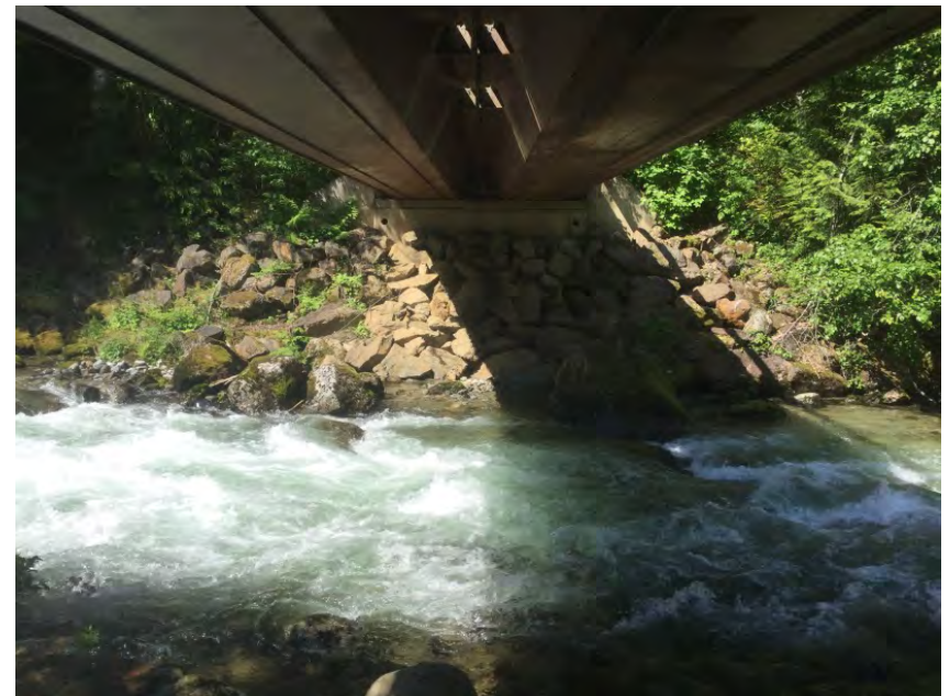
Left Bank Abutment when facing downstream
