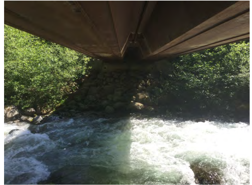
Right Bank Abutment when facing downstream
